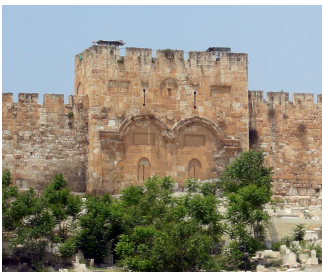
Eastern Gate Sealed Shut
